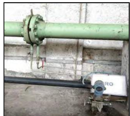
Water meter @Reuse line
