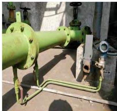
Water meter @Inlet line
