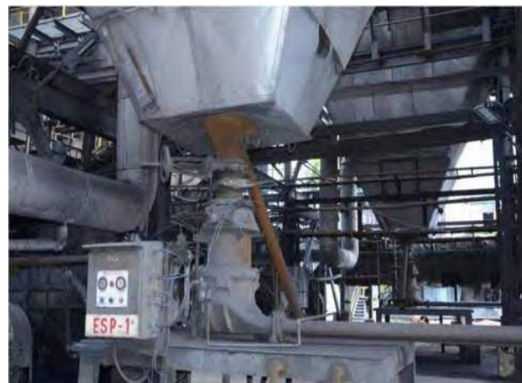
Dense phase pneumatic ash handling system
